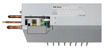
Figure 30: Heat Recovery Unit Control Box With the Cover Removed.
