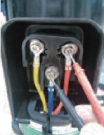
\* Measuring input voltage
