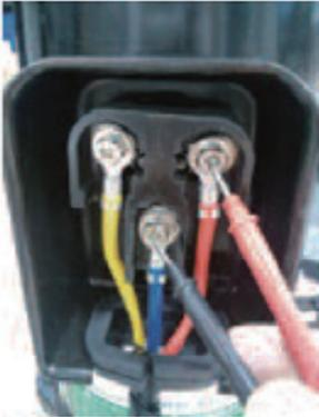
\* Compressor wire connector connection point
